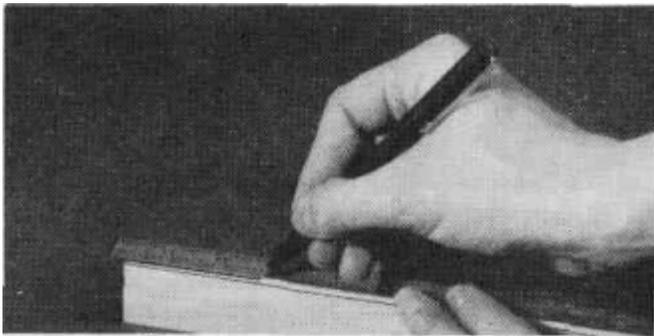
D 6. Remove the elevator and draw a center line down its leading edge. Use your sanding block to sand the same V-shape as you did on the rudder. The trailing edge should also be sanded to a smooth rounded shape.
