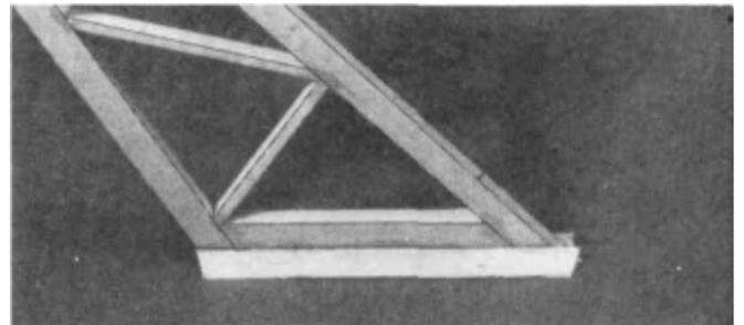
D 5. Cut two 4-1/8" lengths of 3/16" **Balsa Triangle** from SPRTF08 and glue them along the bottom of the fin. The bottom edges of the triangle should be flush with the bottom of the fin.
