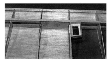
18r. ☐ Place the 1/8" plywood front (larger) sheer web into the groove between the #5 and the #4 rib. DO NOT GLUE AT THIS TIME!
